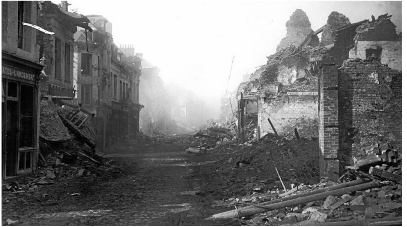
Damaged and burning buildings in Bapaume on March 17, 1917, the day it was occupied by the Australians.
